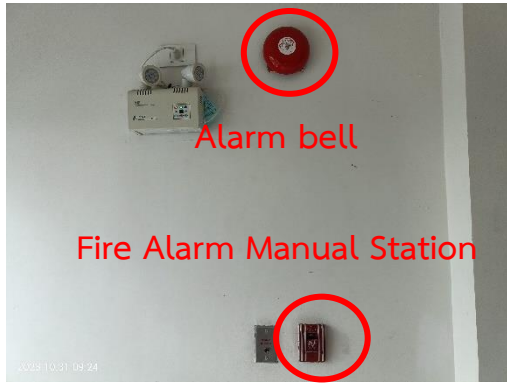
Alarm bell & Fire Alarm Manual Station
