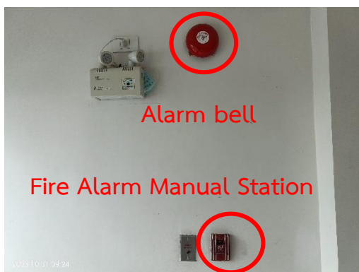
Alarm bell & Fire Alarm Manual Station
